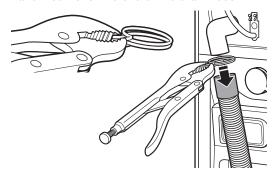
2. Slide the drain hose onto the washer connection.
